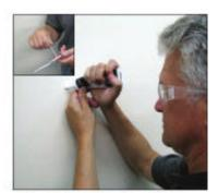
4. Insert the studs into the stud holes on the back of each letter. Place letters in holes on wall <u>before</u> applying silicone to verify position. Adjust as necessary by opening holes with your drill bit. Now fill the drill holes in the wall of the first letter with silicone.
