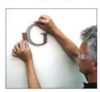
6. Push the letter into the drill holes. If not using spacers, use a thin shim to stand-off slightly from the wall. Secure to wall using long strips of tape. Remove tape after silicone sets. Repeat steps 4 through 6 for the rest of the letters.
