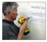
3. Mark holes with center punch, remove pattern if holes are visible on wall, then drill holes <u>slightly larger</u> than stud diameter and 3 inches deep where indicated on your template. Remove the template and clean out all drill holes using compressed air.
